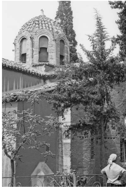
Figure 213 Sotera of Kottakis. Partial view from the southeast.
